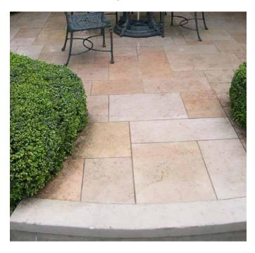
Bush Hammering is a mechanical process that pulverizes the grain of the stone on its surface.
