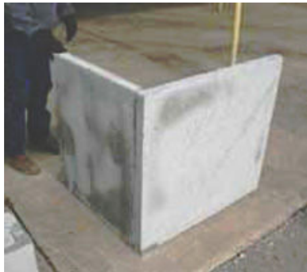
Figure 7. Place Side Panel
