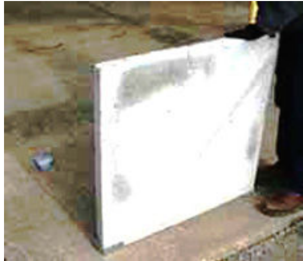
Figure 6. Place Back Panel in Bracket
