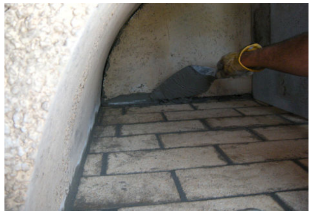
Figure 14. Mortar Inside Joints
