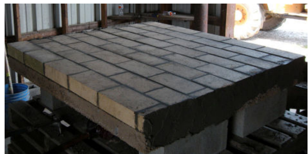
Figure 10. Install Firebrick on Baseplate
