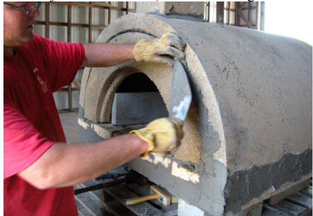
Figure 15. Install Front Wall
