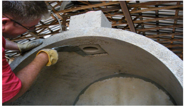
Figure 13. Mortar Chimney Inside of Oven
