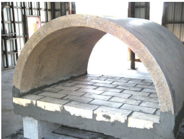
Figure 12. Install Roof
