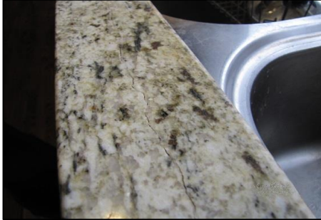
Photo # 99 Blown rod from using metal in wet area and not encapsulated properly (fiberglass preferred)
