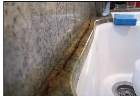
Photo # 60 Blown rod from using metal in wet area and not encapsulated properly
