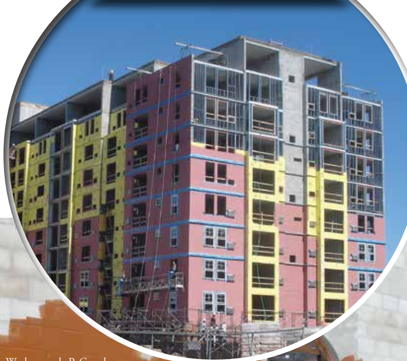
Workers apply R-Guard Spray Wrap on sheathing and concrete blocks.
